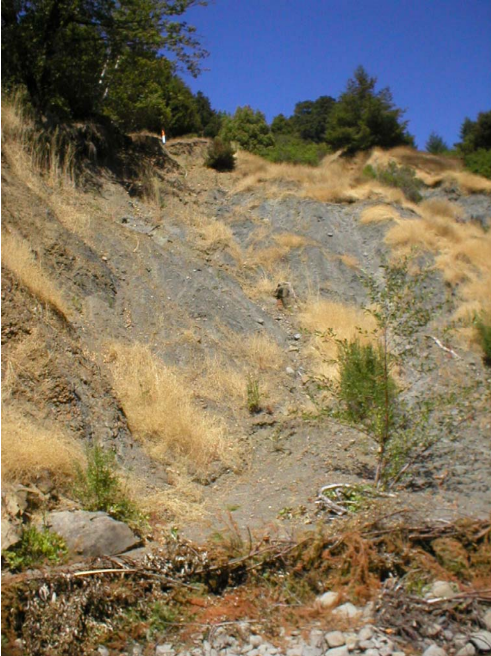
Figure 4. Willow fence at the bottom of Site 27, July 26, 2004.
